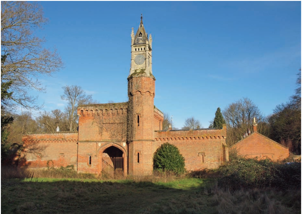
FIG. 163 – The entrance to the stable block with the clock tower on its right, and the low electricity generating house on the extreme right.
