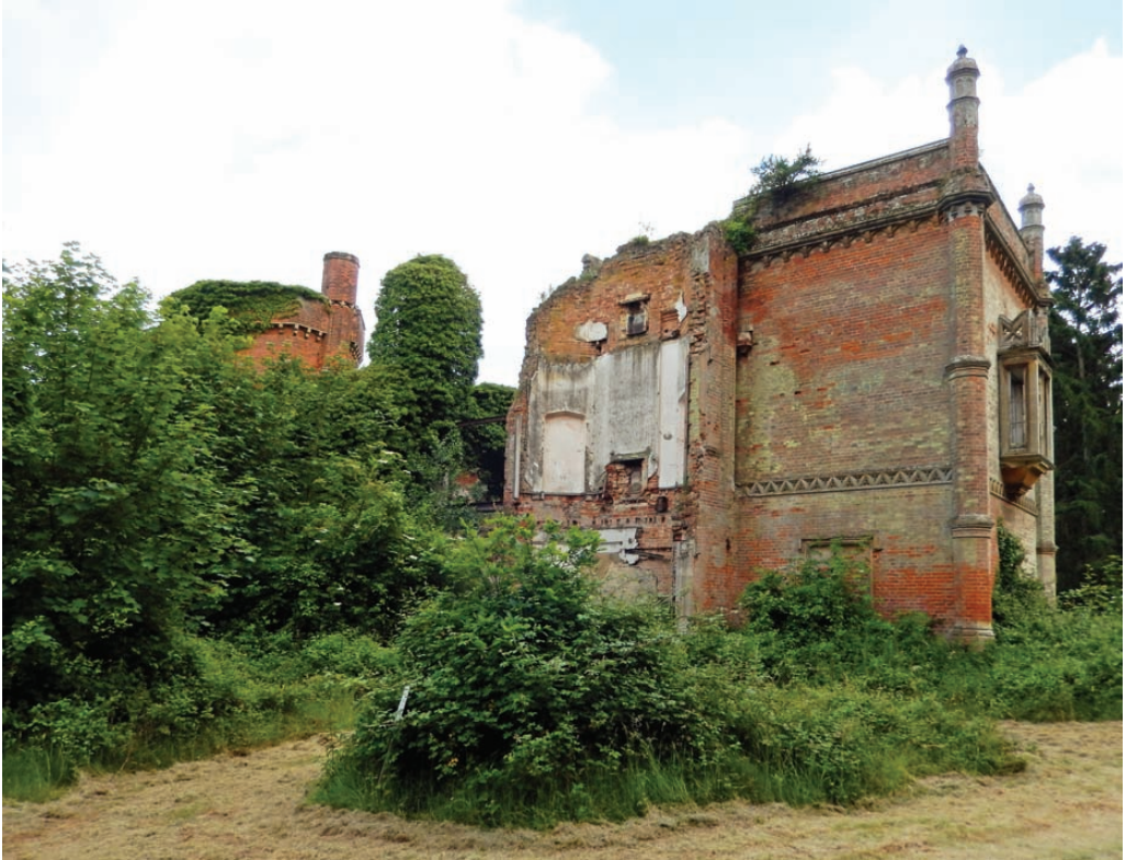
FIG. 164 – North side of Rougham Hall showing the damage caused by the German bomb in 1940 and the eventual demolition of the West Tower in the 1970s. The exposed room was a bedroom, with another more fragmentary one above it, both over the entrance hall. The surviving section to the right contained the drawing room, with a bedroom with an oriel window above it. The East Tower, in the background, contained the boudoir, with ‘Mr Agnew’s Dressing Room’ above it, and a bedroom above that.
